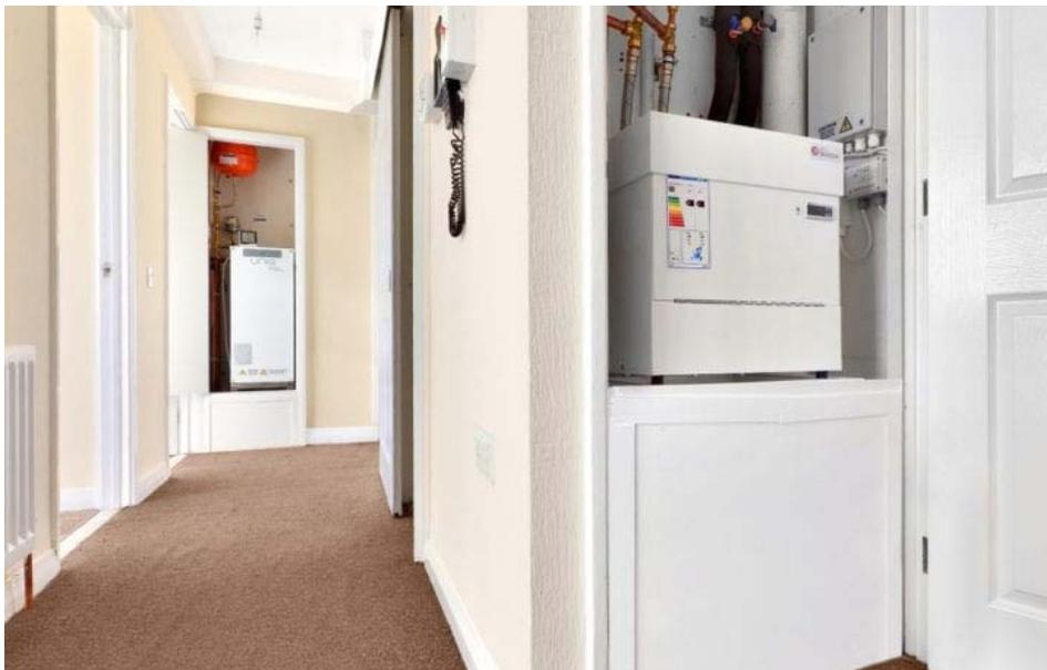
Photo 7: A Kensa 3kW 'shoe box' heat pump (photo courtesy of Kensa Contracting)
