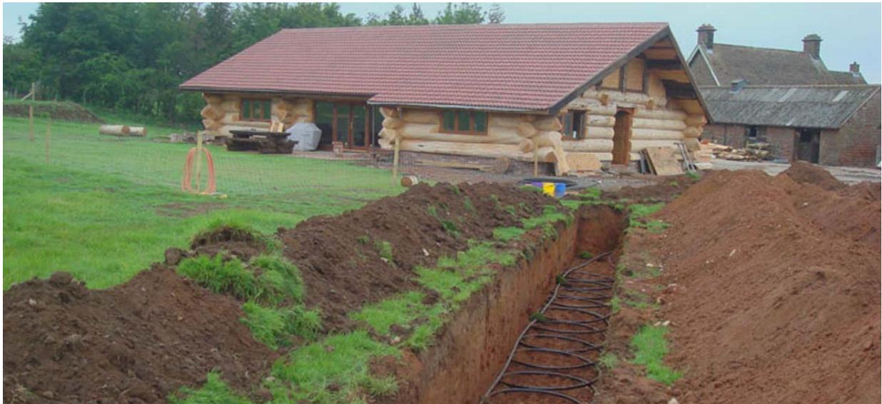
Photo 2: Horizontal ground loop (courtesy of CA Heat Pumps Ltd)
